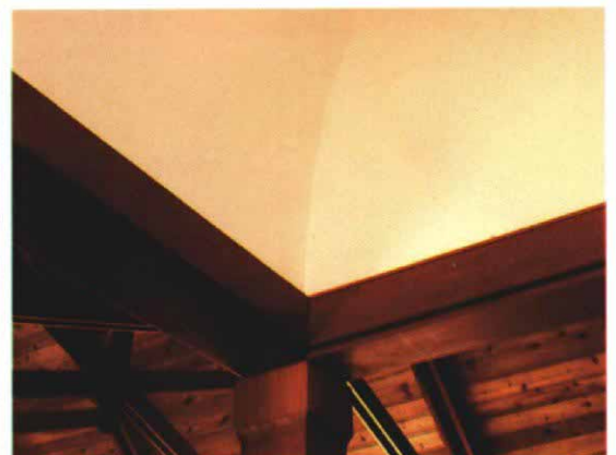
An inside corner of the coved ceiling. Curved ribs were cut from 2x12s, as at left. These ribs were covered with expanded metal lath, the base for three coats of plaster.
