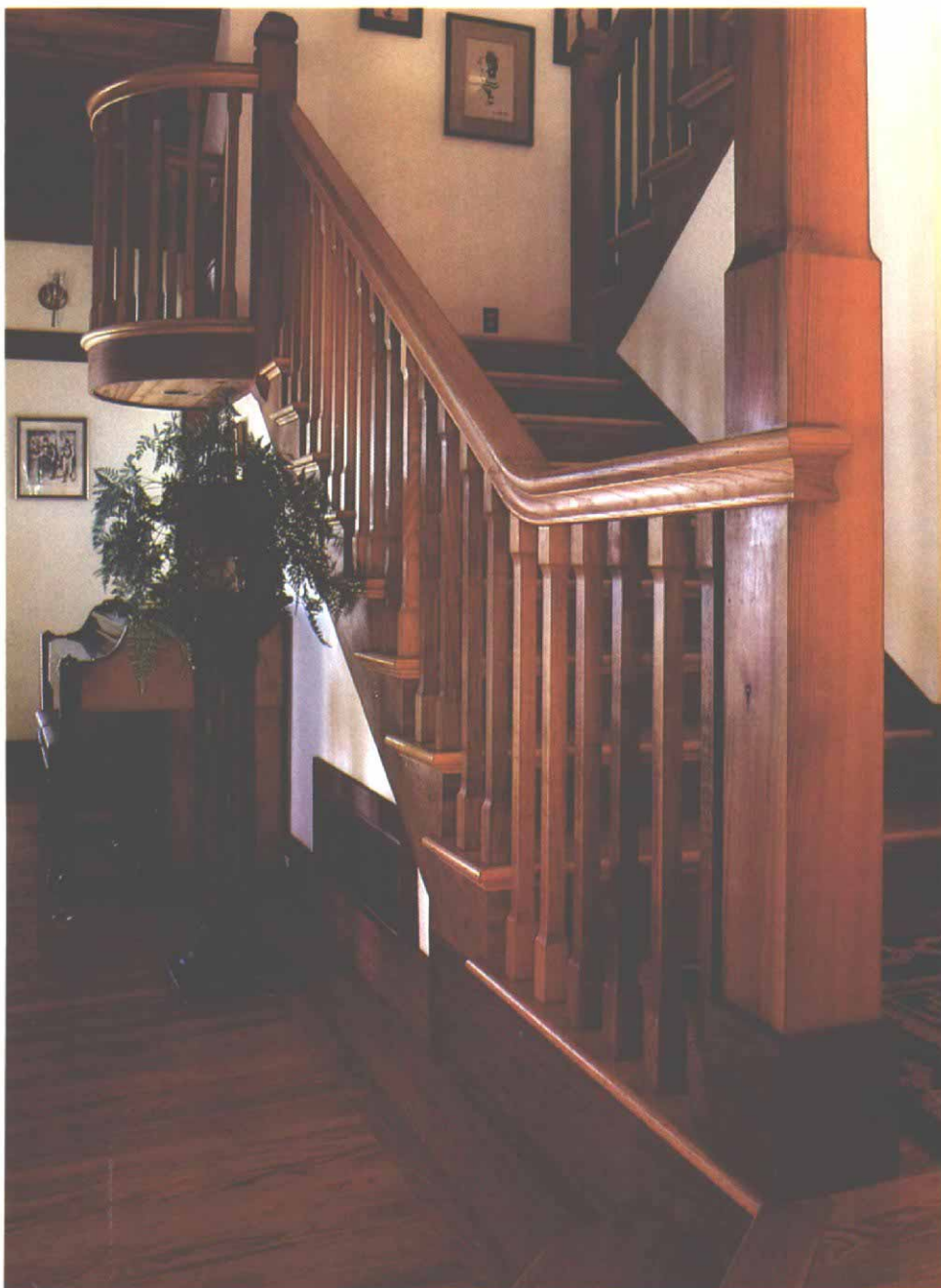
It took two men 230 hours to build and install the stair. The handrail is red oak; its side pieces were coved out on a table saw, and the balusters were shaped from 2x cedar stock.
